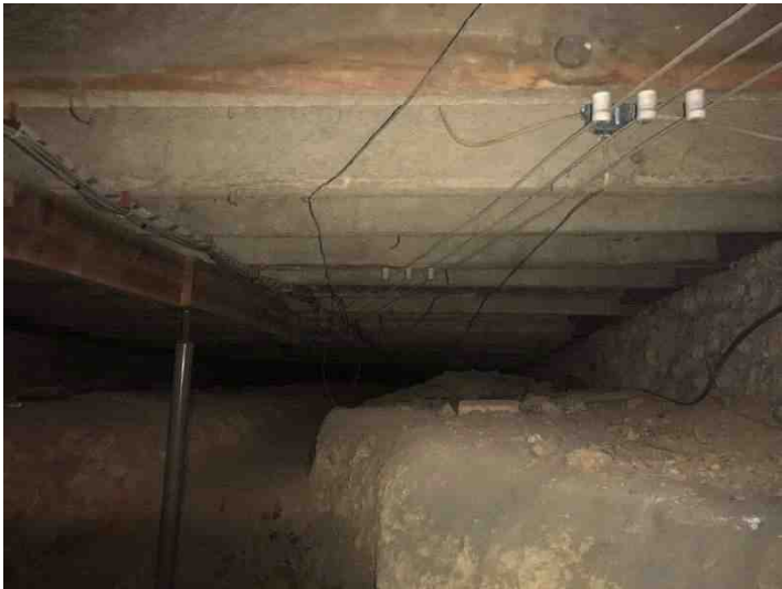
crawlspace and knob/tube wiring under sanctuary
