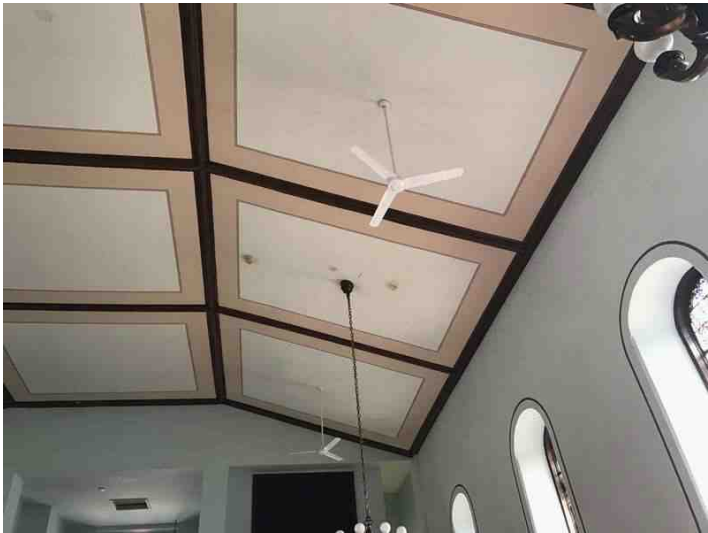
stain on ceiling from past leak, roof was replaced two year ago
